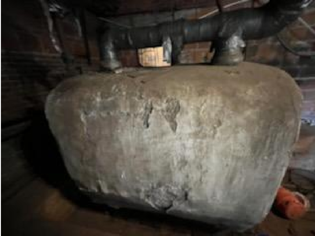
View of ACM Insulation on Boiler
