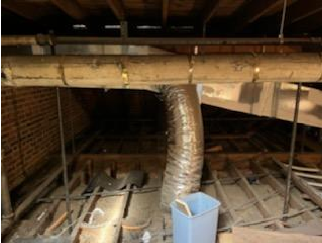
View of Pipe Insulation ACM
