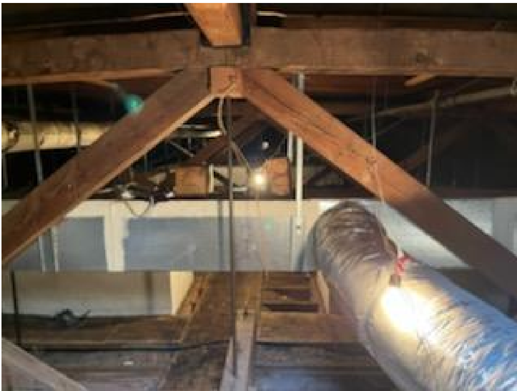
View of Pipe Mastic ACM
